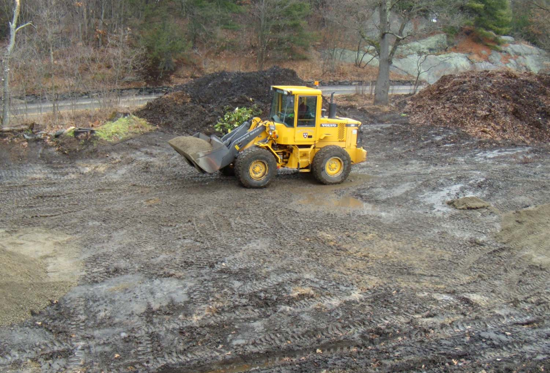
FMO Composting Facility under construction at the Arnold Arboretum. November 2008
